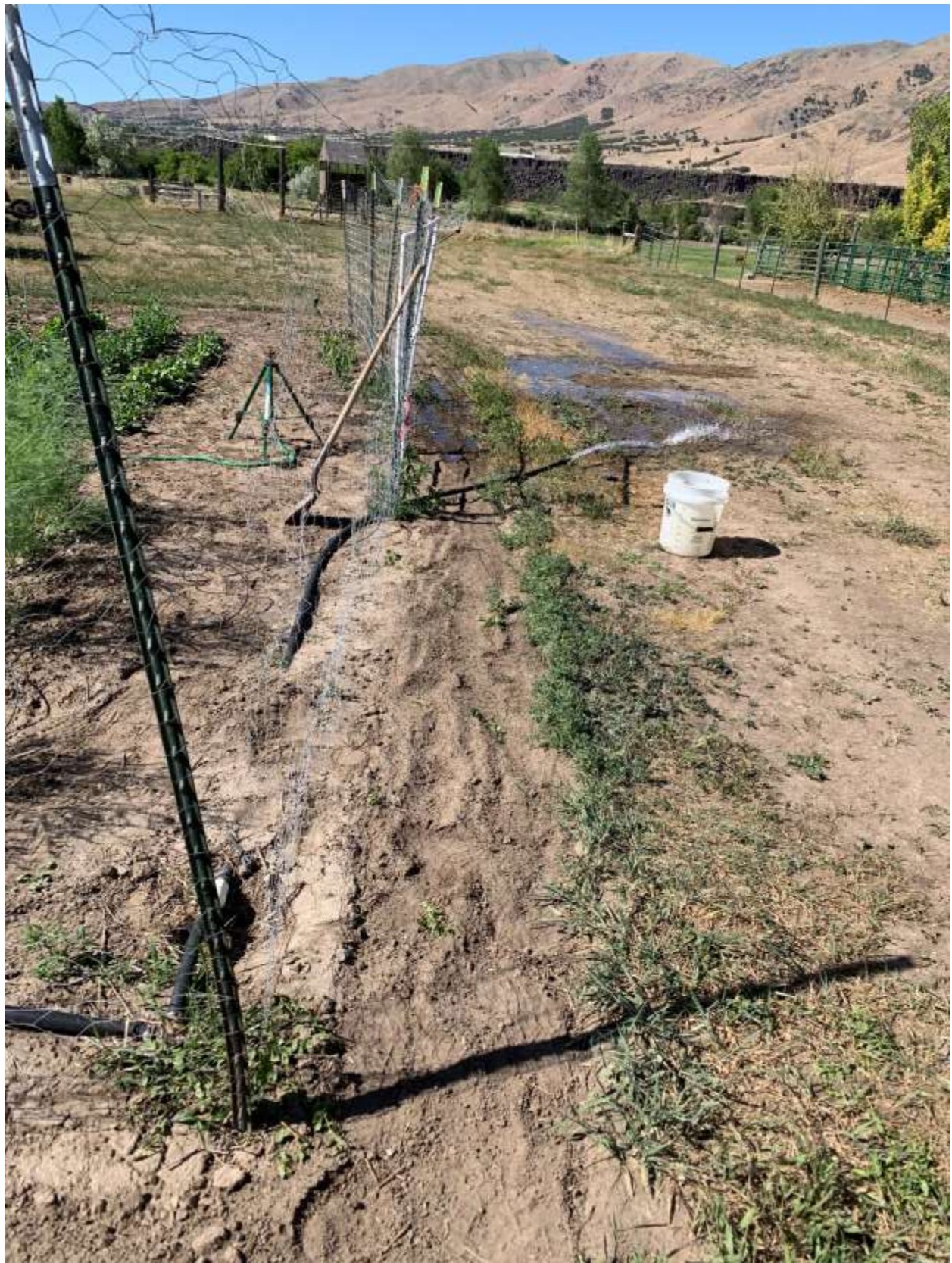
RW-7586P Conveyance Line 06/21/2021
