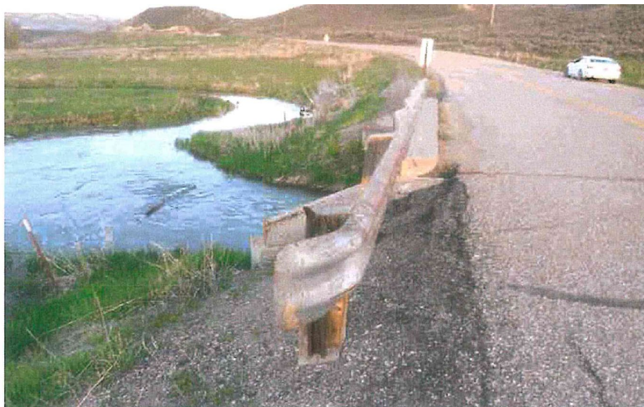
Guardrail Ends - Narrow Shoulder on Bridge
