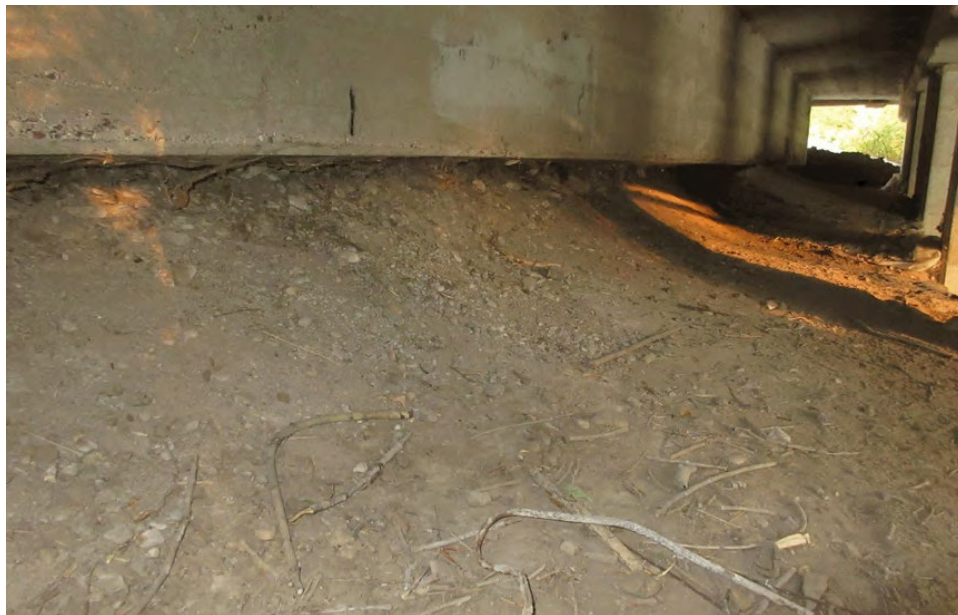
Figure 11 – North cantilevered bridge end: the concrete is undermined.
