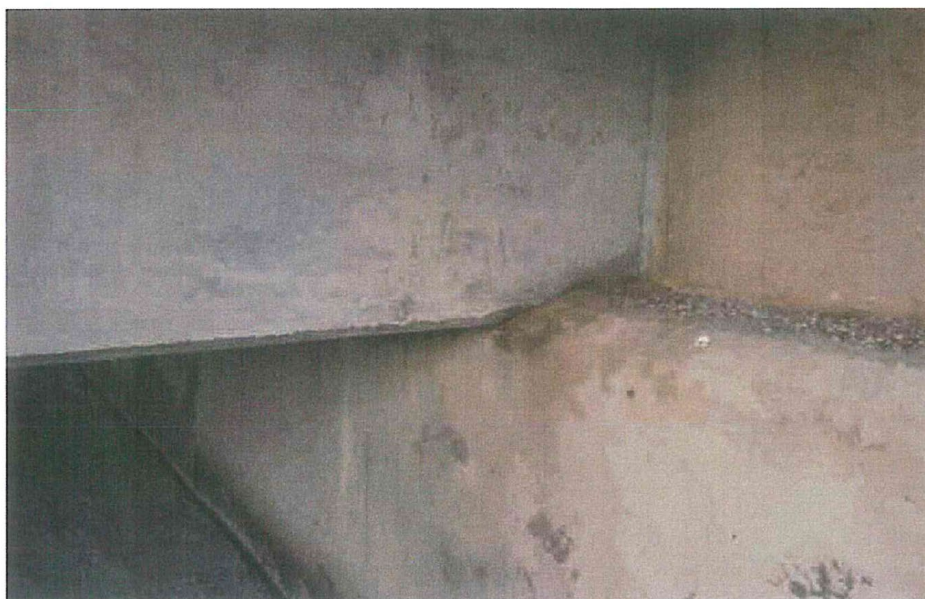
Bearing - Directly on Concrete
