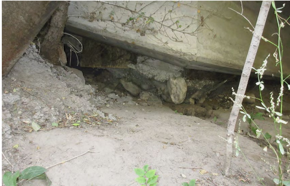
Figure 10 – South cantilevered bridge end, east side: the end concrete is undermined.
