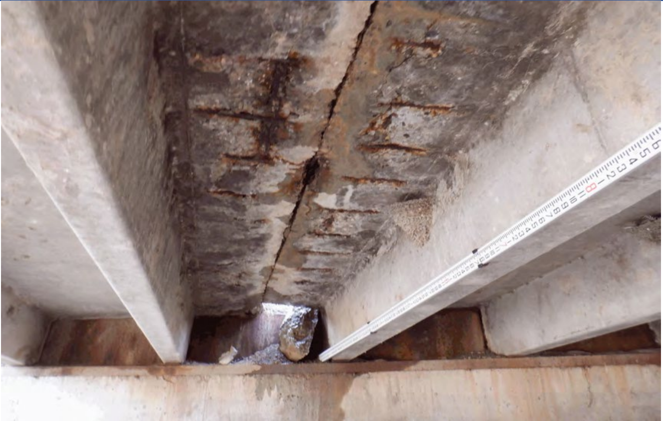
Figure 9 – South Girder Joint Corrosion and Spalling – Looking West
